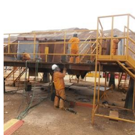
On-site maintenance and shutdown services (Pilbara Hire)
