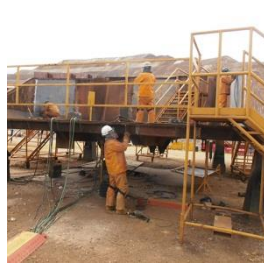
On-site maintenance and shutdown services (Pilbara Hire)
