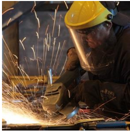
Equipment repair and maintenance
